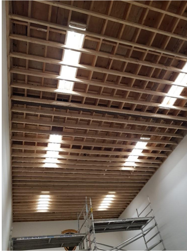
Fig 15.0 – Installation for Ceiling Joists
