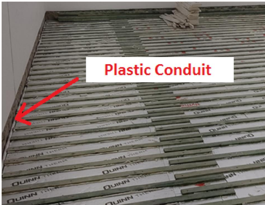
Fig 6.0 – Plastic conduit around perimeter of alley
