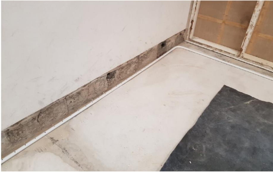
Fig 5.0 – Installation of 25mm Plastic Conduit
