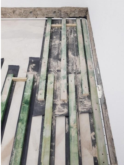
Fig 3.0 and 4.0 – 3"*2" Batten installation
