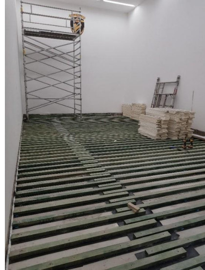
Fig 3.0 and 4.0 – 3"*2" Batten installation
