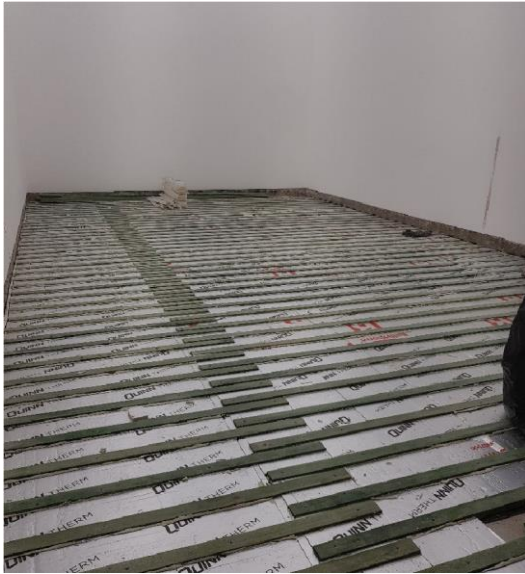
Fig 1.0 – Installation of 25mm Floor Insulation
